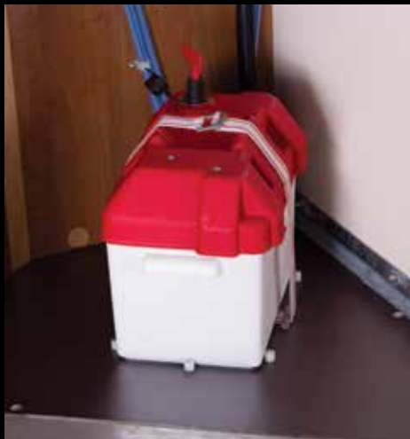
On board 12v electrics
